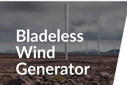
The latest development in wind turbine design isn't a turbine. In fact, it has no moving parts at all! The simple design – which resembles a giant straw – means that it's less expensive to manufacture, cheaper to maintain, and should last considerably longer than typical wind turbines.
