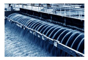
oxygen concentration of about 2 milligrams per liter. It has long been believed that this was necessary to keep the microorganisms alive and working at an optimum level. However, it was found that lower concentrations (about 0.5 milligrams per liter) produced the same results while using about 30 percent less energy. In addition, the microorganisms lived longer and enriched more.
