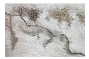
The protective coating is designed to be sprayed on the surface, preventing small surface cracks from developing into larger ones that could compromise integrity of the structure. When small cracks appear, polymer microcapsules release their contents – a solution that turns into a water-resistant solid when exposed to light and protects the underlying concrete from further damage.
